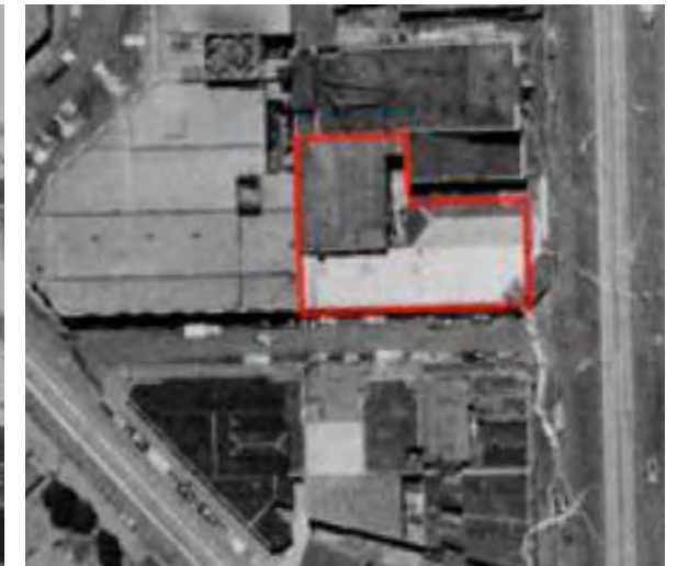
1946 Aerial photograph of site
