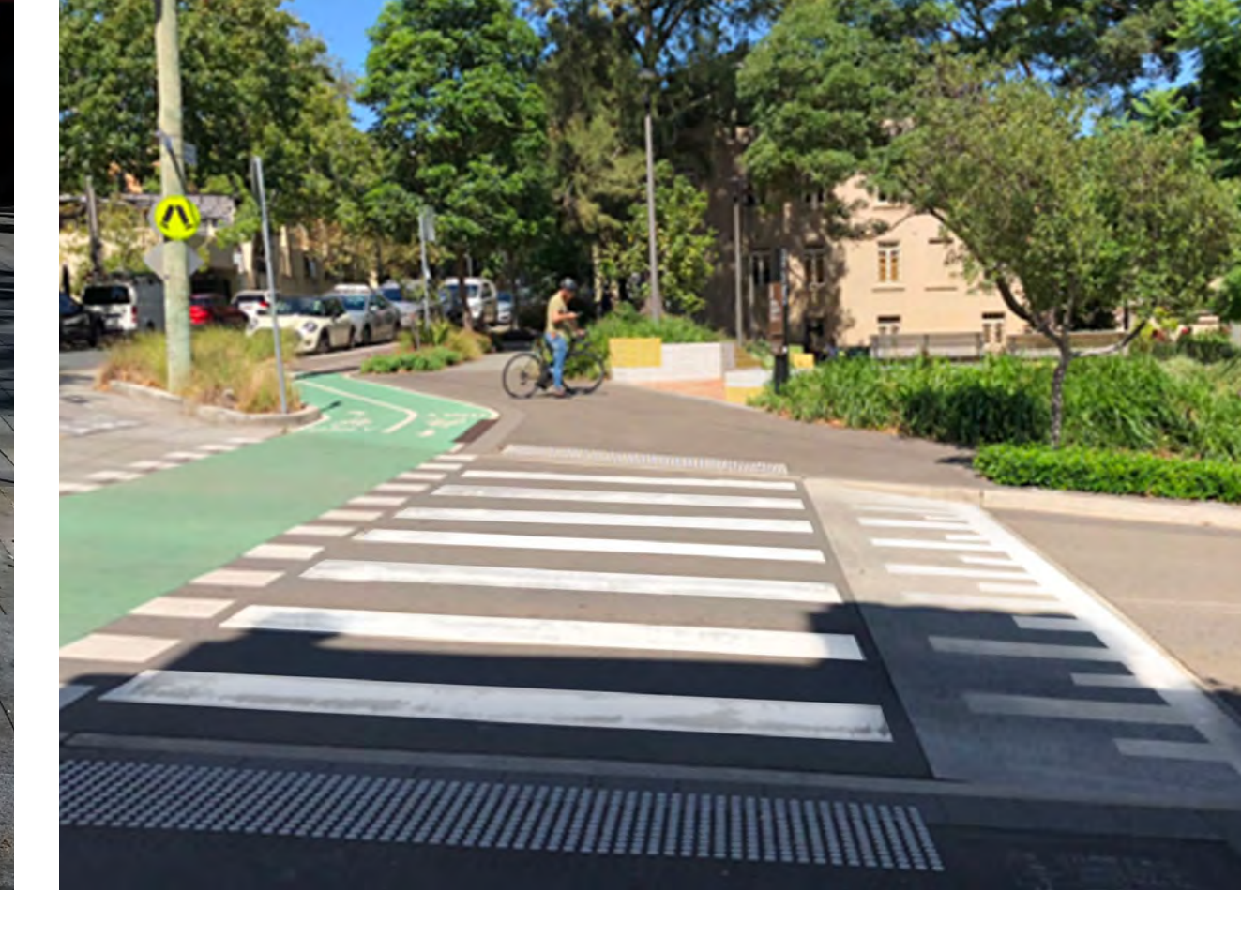
pedestrian crossing with adjacent bike crossing
