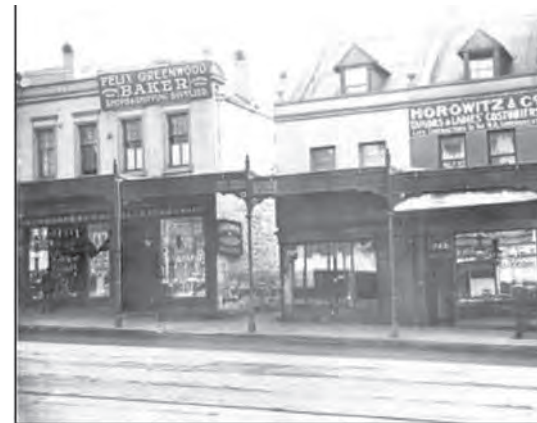
1910, access lane in approx. location of proposed cross site link
